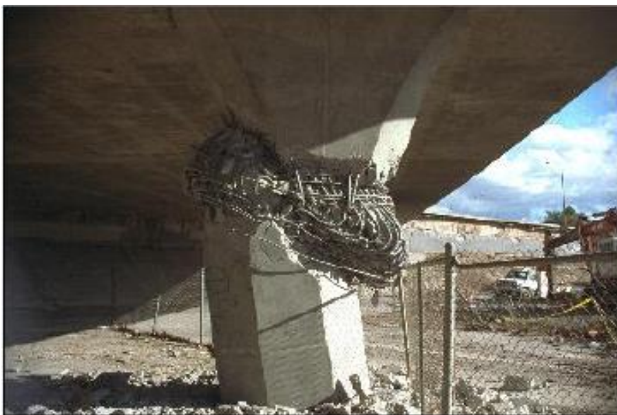
Appendix Figure A-8 - - Earthquake Damage (Source: FEMA)
